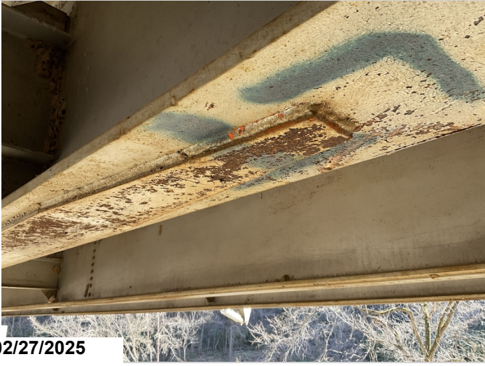
Cover plate welding detail. This is an E detail.
