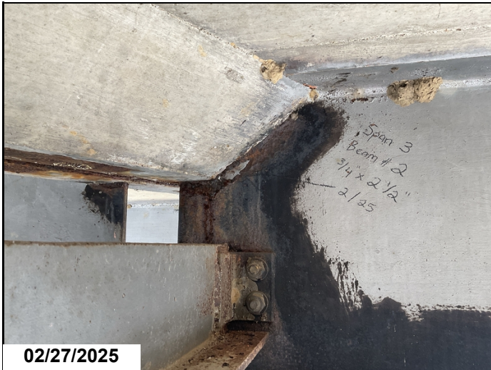
02/27/2025 3/4" tall by 4" long rust hole in the upper web of beam #2 at the beginning of span #3.
