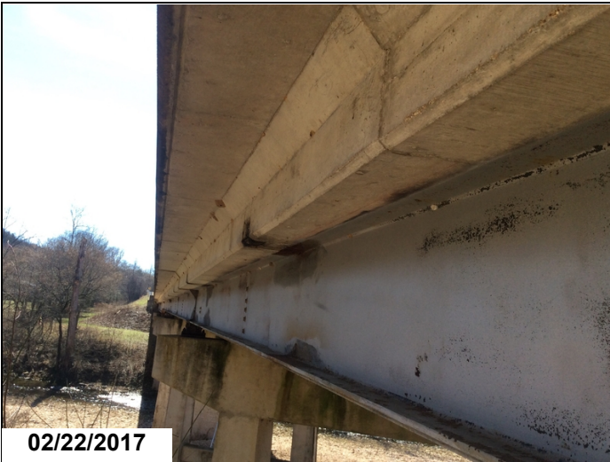
Corrosion beneath drains along the left and right sides of structure.
