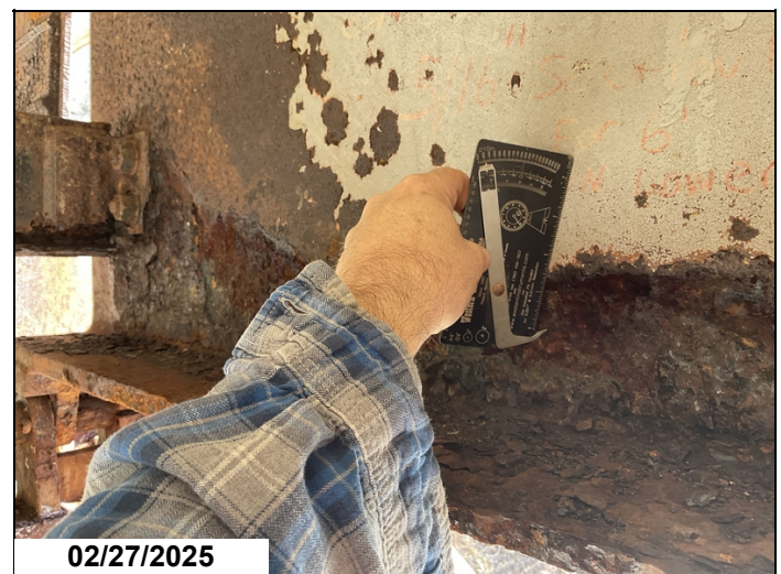
02/27/2025 3/4" tall by 4" long rust hole in the upper web of beam #4 at the beginning of span #3.
