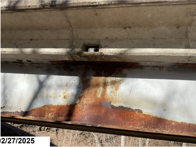
Area of cs3 corrosion on the exterior beams beneath the drain areas. Typically 3' long with up to 1/4" deep section loss.
