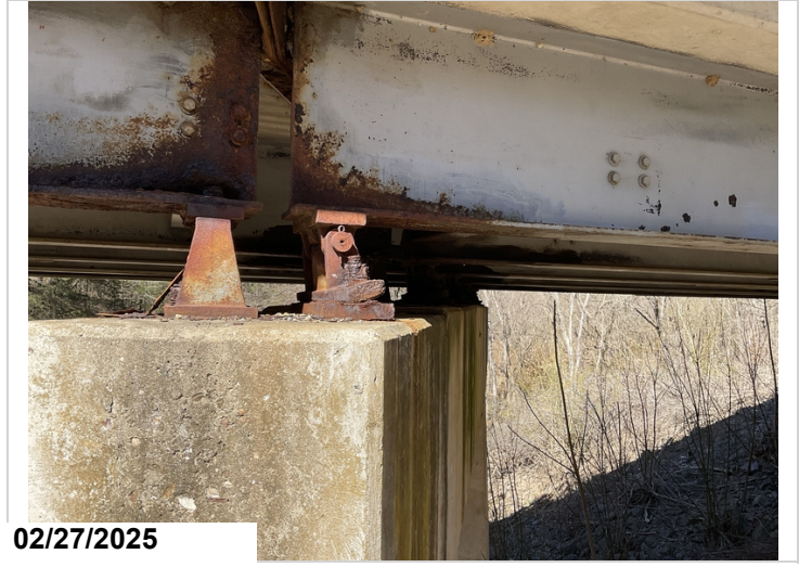
The moveable bearings at pier #4 span #5 are all tilted toward span #4.
