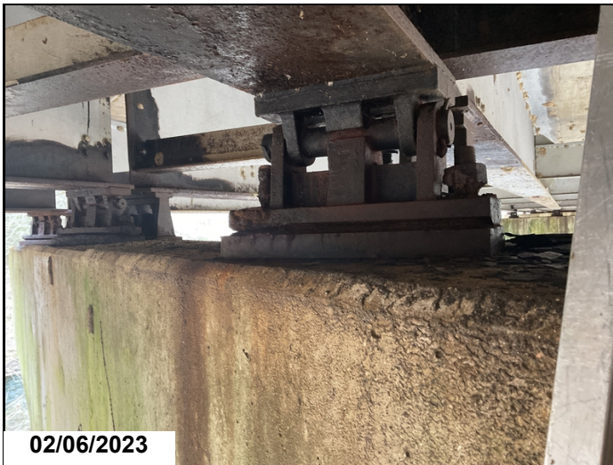
Anchor bolt section loss and bearing corrosion over pier #1.
