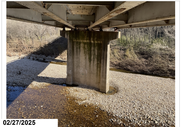
Typical view of the bents with web wall.
