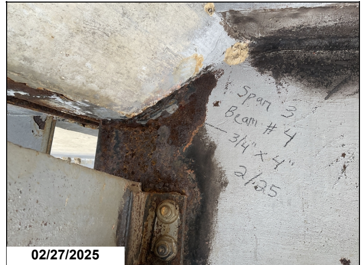
02/27/2025 3/4" tall by 4" long rust hole in the upper web of beam #4 at the beginning of span #3.
