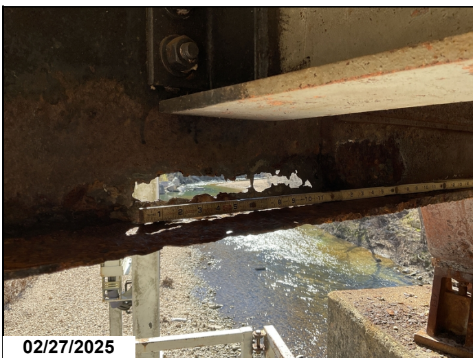
02/27/2025 3/4" tall by 4" long rust hole in the upper web of beam #2 at the beginning of span #3.
